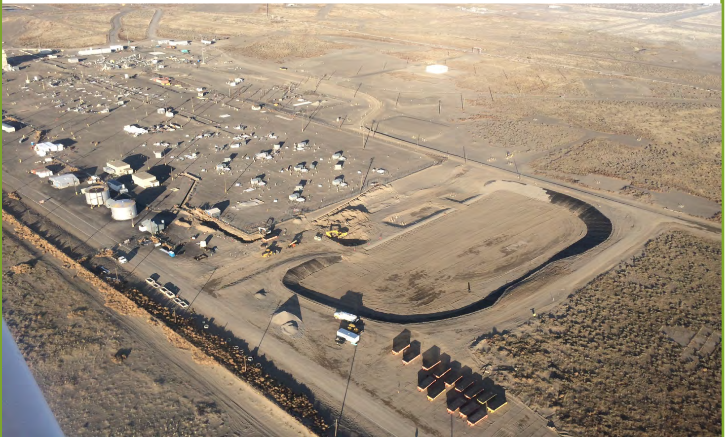
Aerial view of SX farms and evaporation basin
