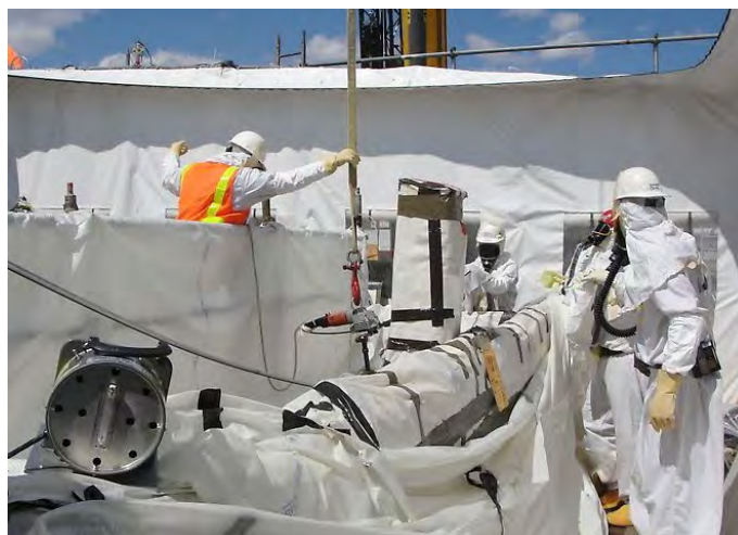
Workers preparing equipment in the tank farms.
