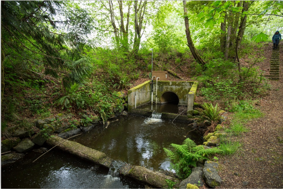
Figure 21. Culvert and weir system on Springbrook Creek just downstream of Fletcher Bay NE.
