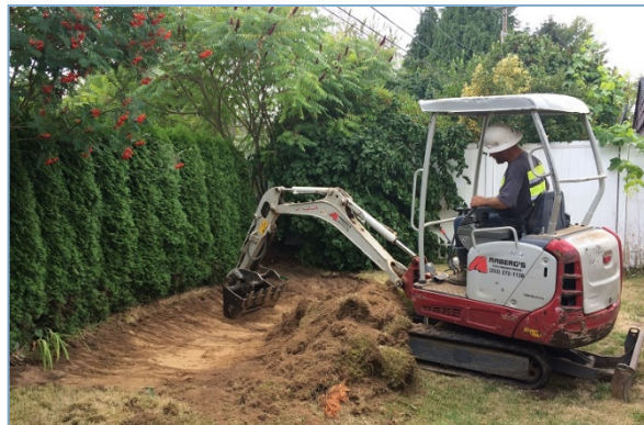
Photo 3: Contractors removed the top 18 inches of contaminated soil at a home in Tacoma.
