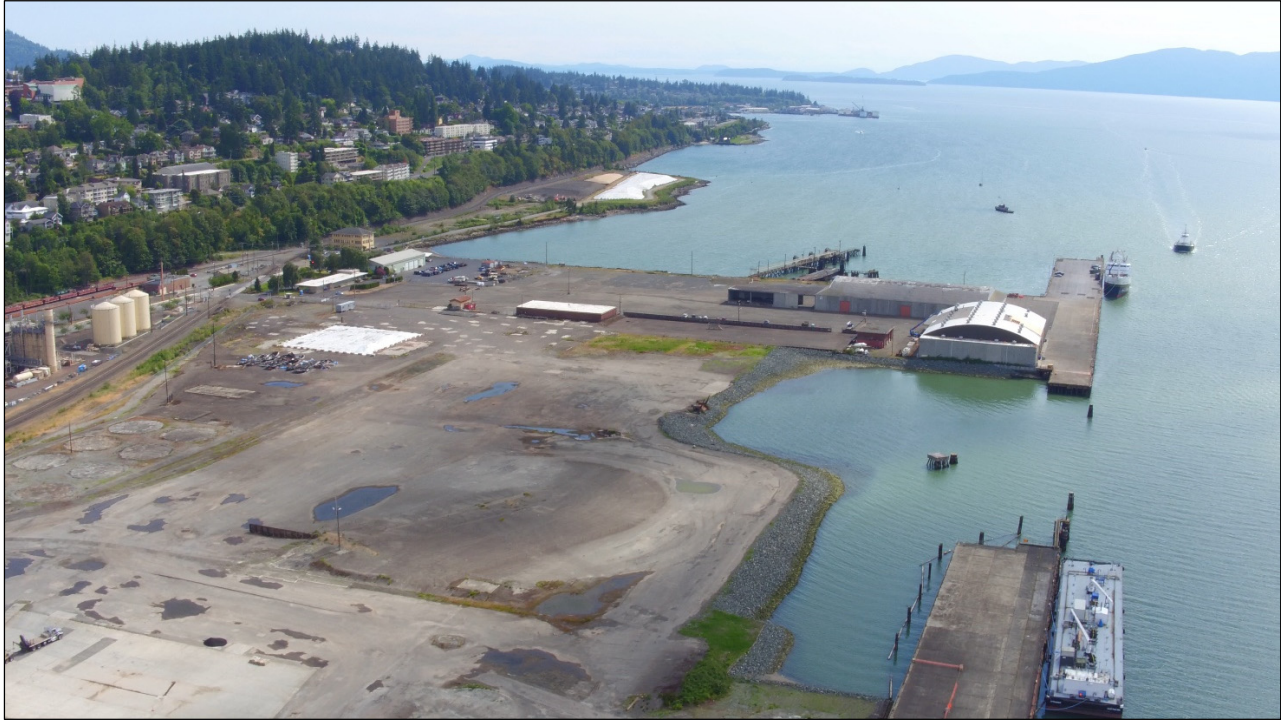
Georgia Pacific West Site, Chlor-Alkali area facing southwest. November, 2016.
