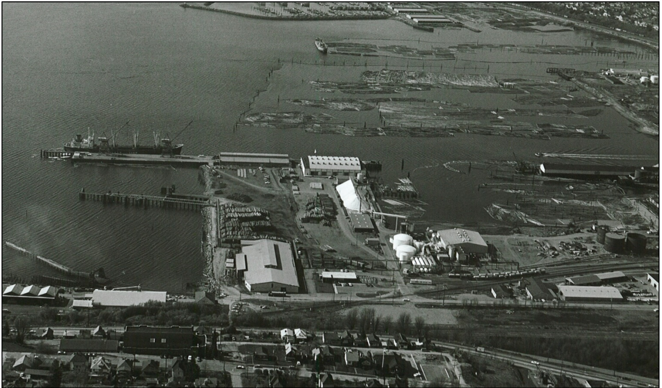
Georgia Pacific West Site, Chlor-Alkali Area facing northwest, 1969.
