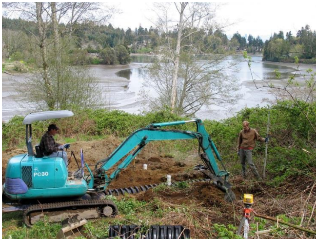
Figure 1: An excavator installs a new drainfield.
