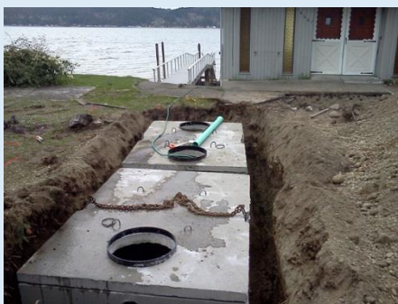
Figure 3. New septic tanks.
