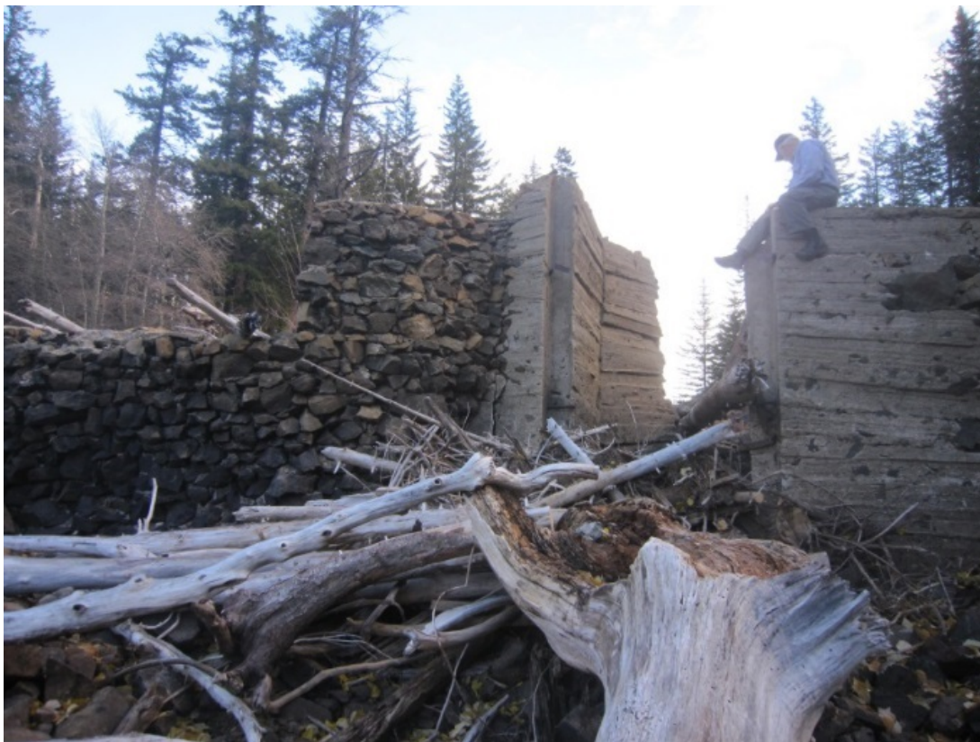
Figure 2-20. Current Alpine Lakes Infrastructure, Eightmile Dam (2015)
