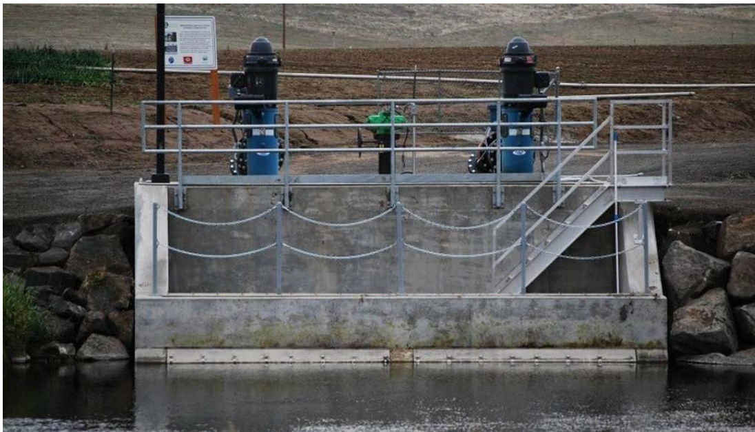
Figure 4-49. Representative Photo: Pump Station Intake Features and Armored Bank
