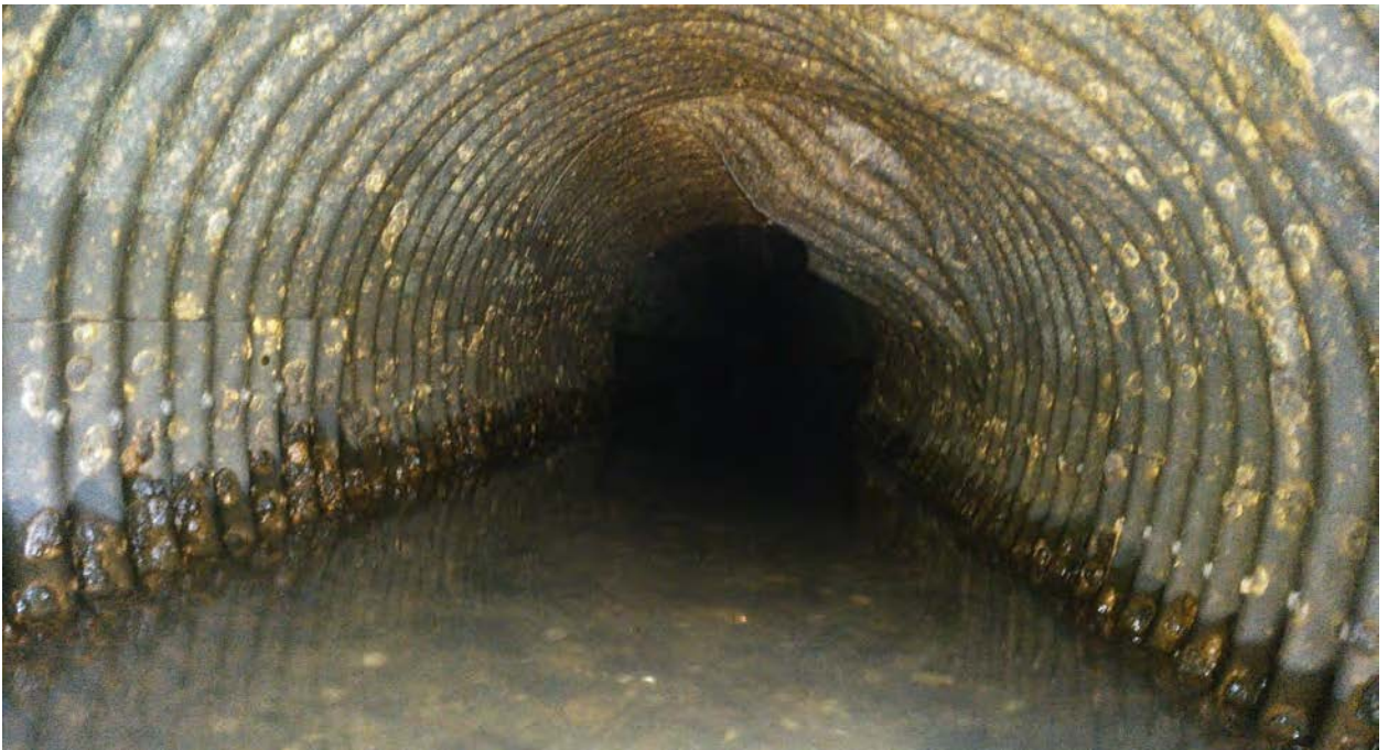
Photograph 11 Low-Level Outlet Pipe, Near Pipe Outlet
