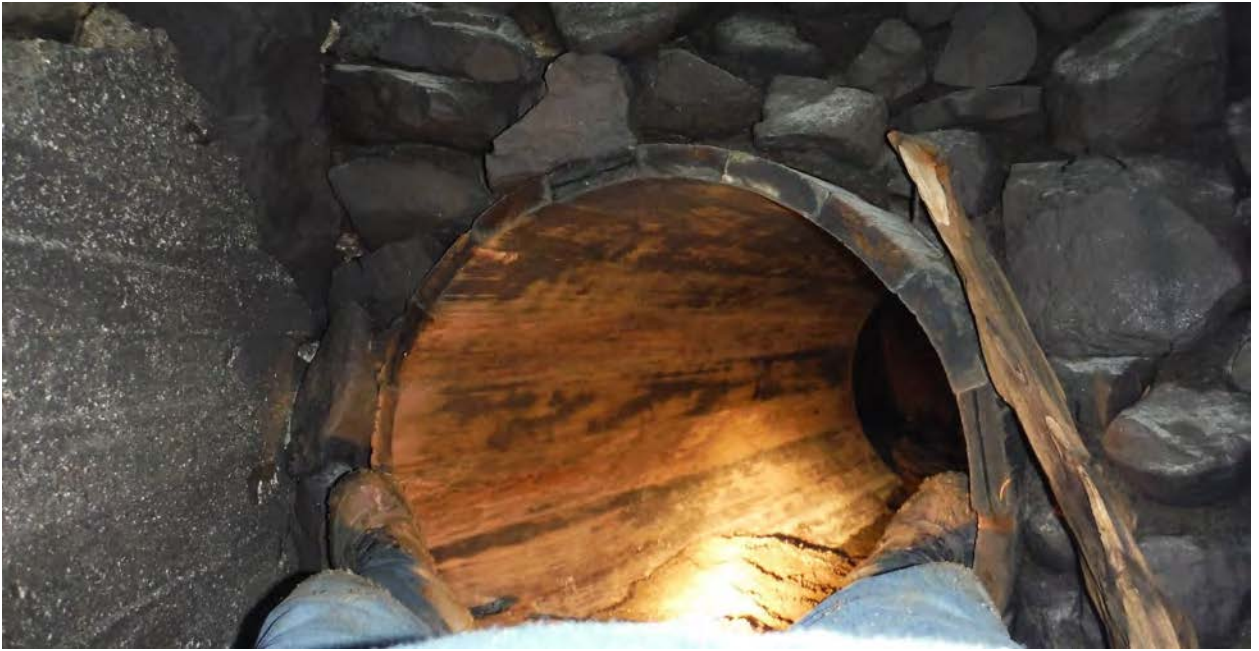
Photograph 10 Low-Level Outlet Pipe, Wood-Stave Section
