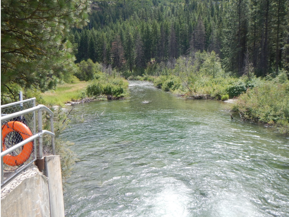
Figure 4-23. Icicle Creek Viewpoint 2: From Structure 2 Looking Downstream (Mid-water, 390 cfs)
