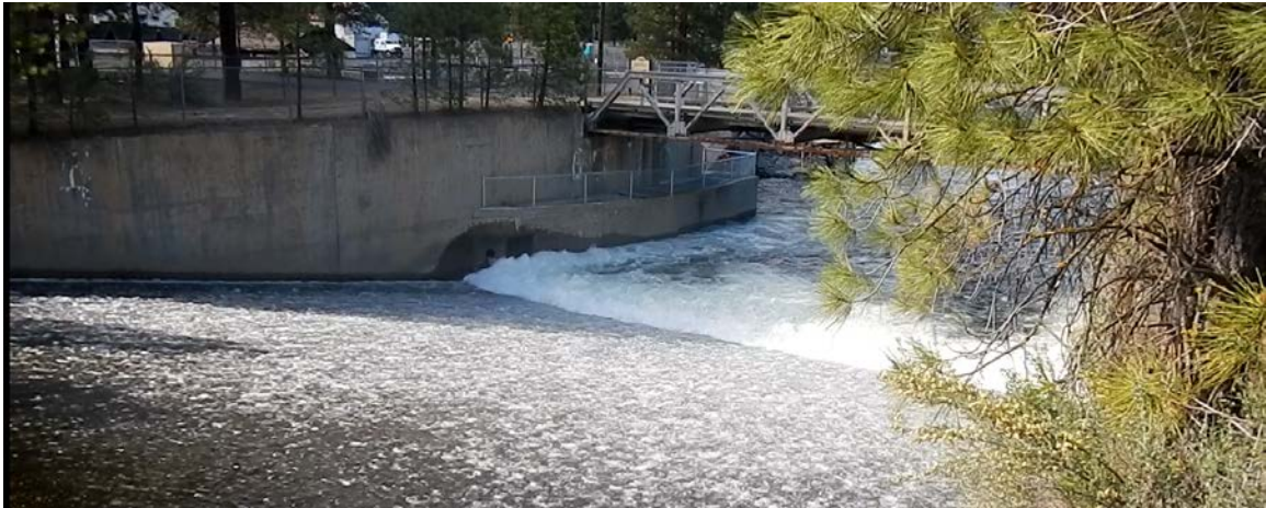
Figure 2-33. 1,700 cfs at Plunge Pool
