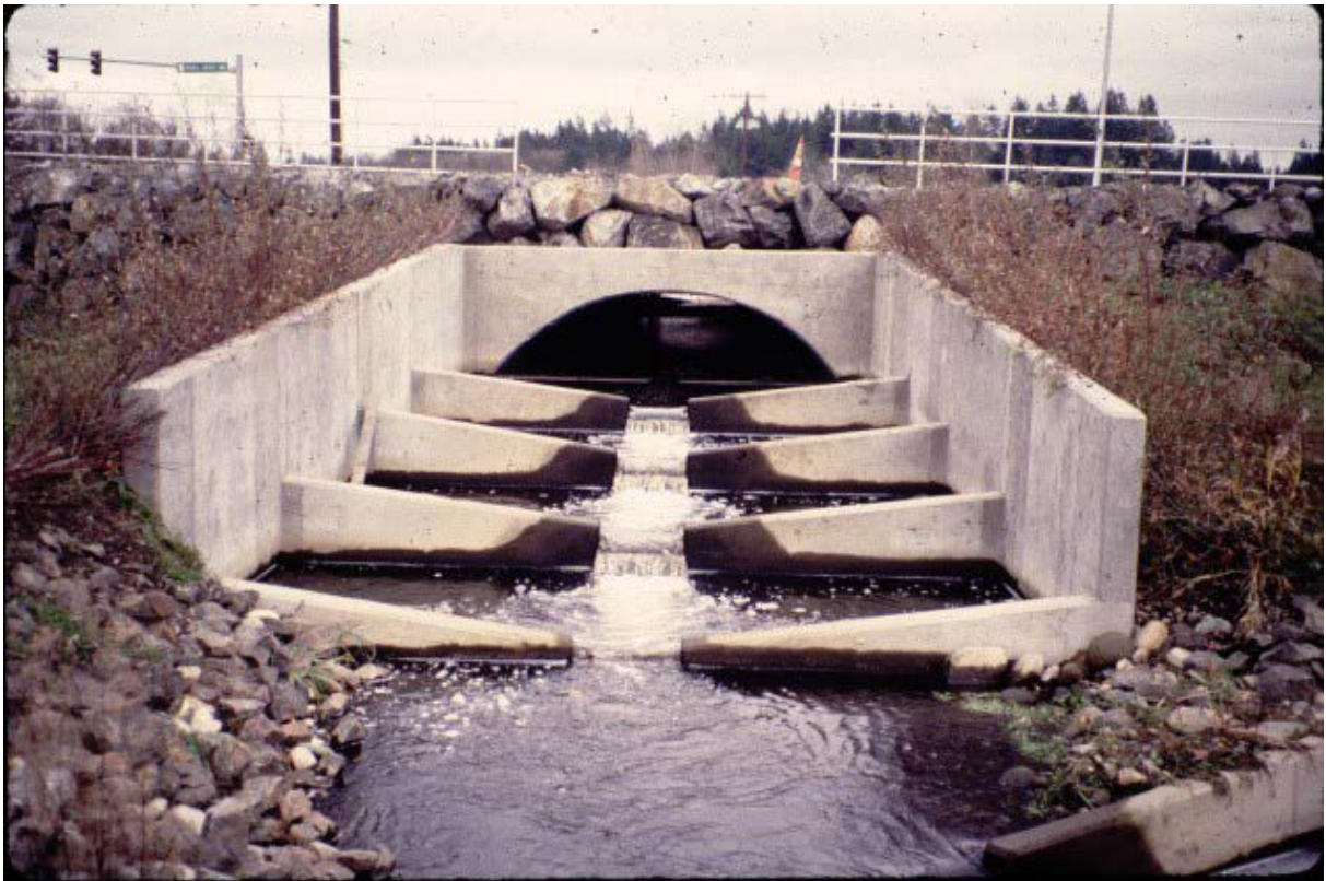
Figure 2-42. Example of pool and chute fishway
