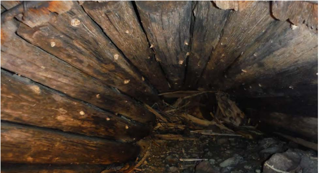
Photograph 9 Low-Level Outlet Pipe, Log-Stave Section
