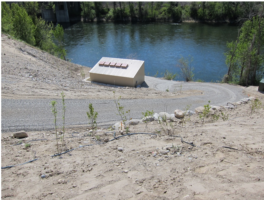
Figure 4-50. Representative Photo: Pump Station Building (Prior to Revegetation)
