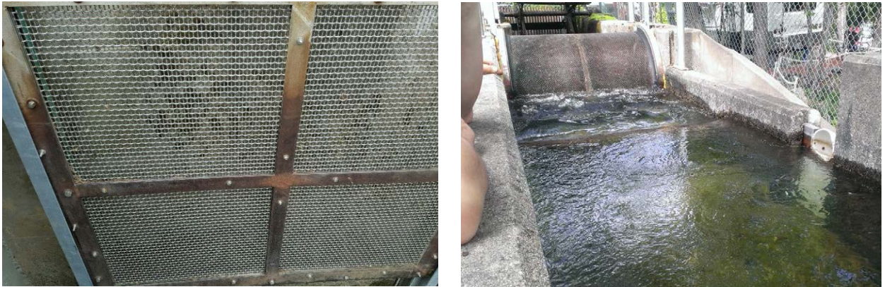
Figure 2-43. LNFH/COIC Fixed Plate Screen (left) and COIC Bypass Screen (right)
