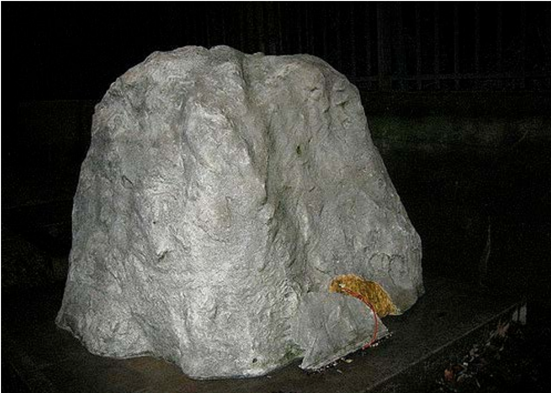
Figure 28 – Representative Photo: Utility Cover
