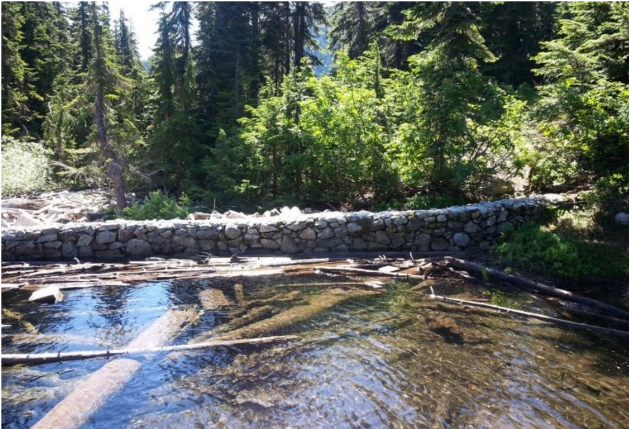
Figure 2–24. Current Alpine Lakes Infrastructure, Square Lake Dam
