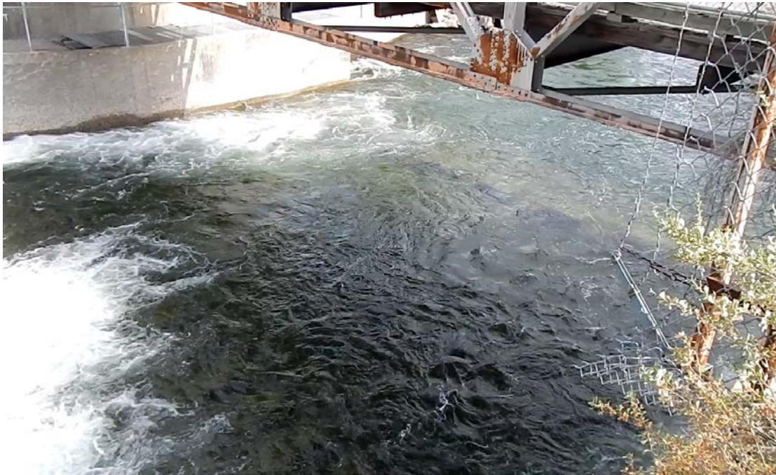
Figure 2-32. 700 cfs at Plunge Pool
