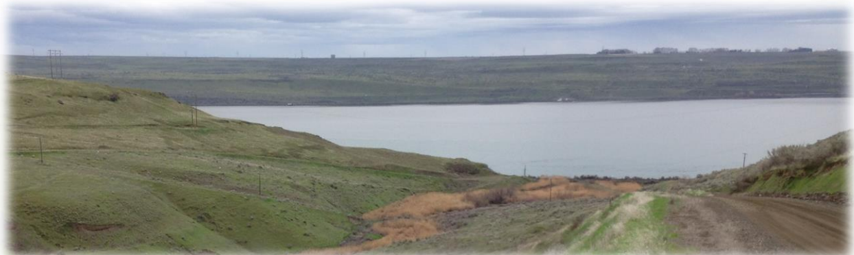
Proposed Switzler Reservoir Storage Project Site
