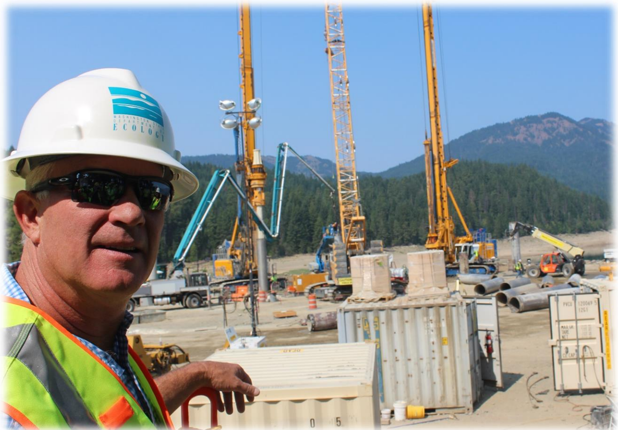
OCR's Director, Tom Tebb, at the Cle Elum Fish Passage construction site
