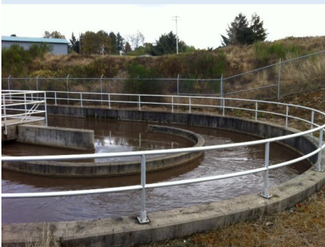
Figure 6: Flood prevention dike along Pe Ell's wastewater treatment plant.
