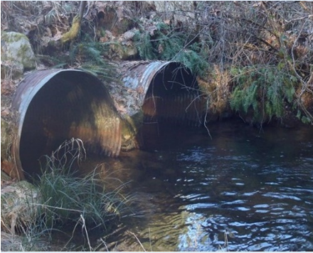
Figure 8: These Bush Creek barrier culverts are being replaced.
