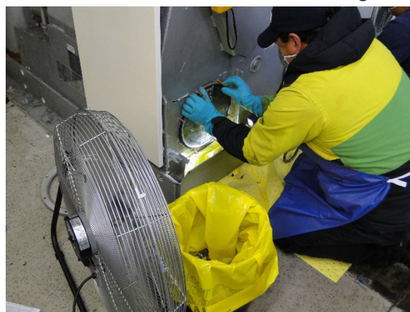
Figure 1. Box fans set up to remove PERC vapors. Photo by Stephen G. Whittaker, King County
