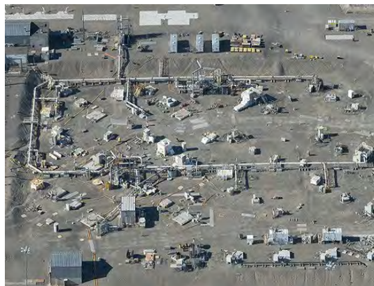
Now that retrieval is complete, much of the support infrastructure has been removed. (Courtesy DOE)
