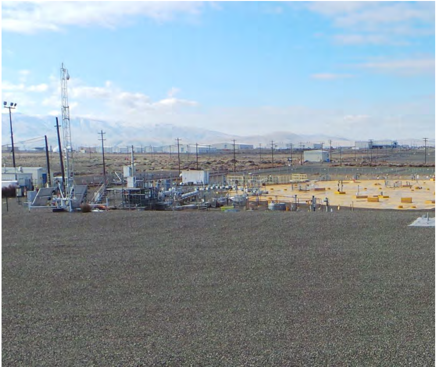
Tank T-111 is located in the T Tank Farm in the 200 West Area of the Hanford site. The yellow portion is the 241-T interim barrier.
