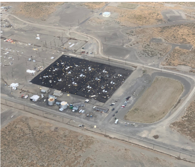
Figure A. Features seen on the interim barrier provide access to tanks and infrastructure beneath the barrier. These features are capped to prevent moisture from seeping through the barrier into the soil and water table below.
