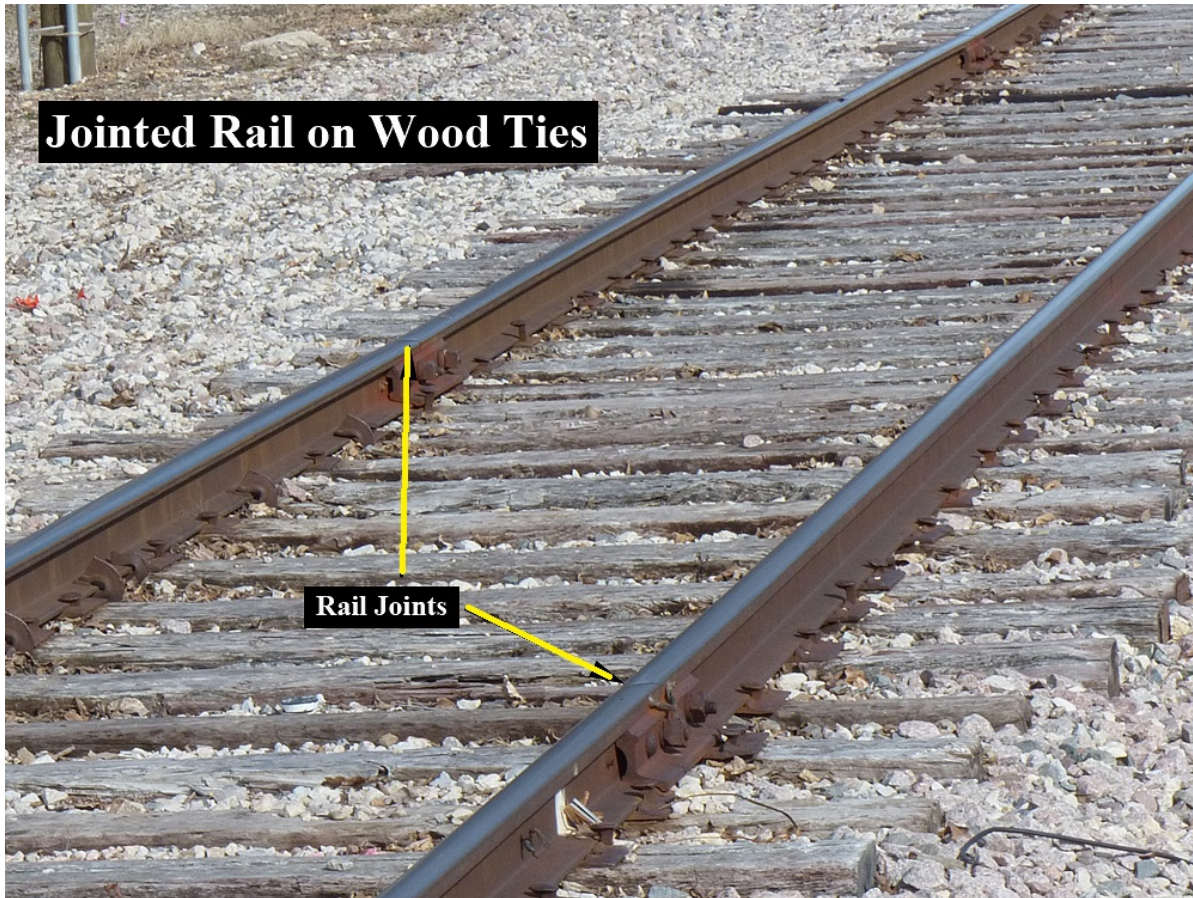
Figure 110: Jointed Rail on Wood Ties Showing Rail Joints 437
