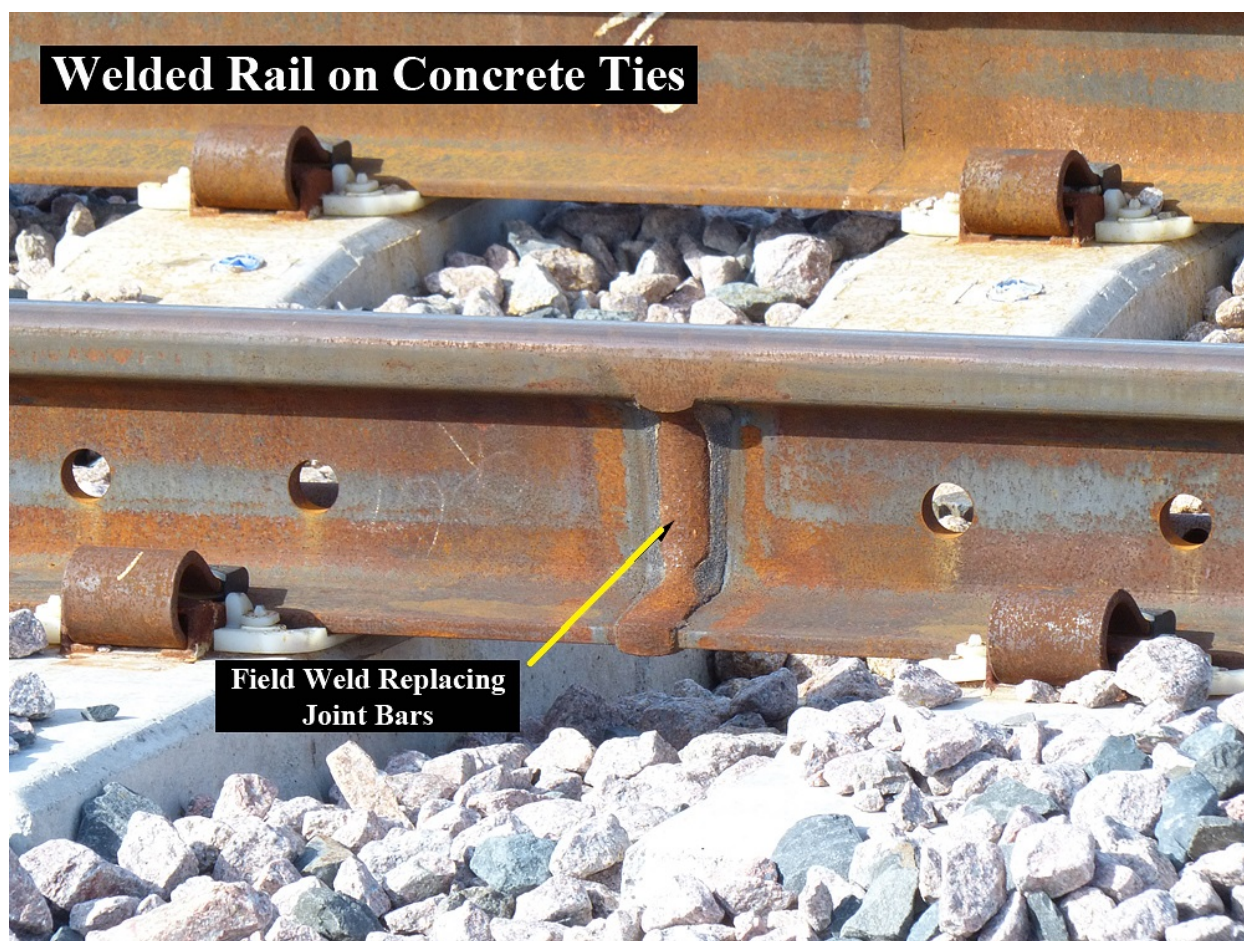
Figure 72: Welded Rail on Concrete Ties (Field Weld Replacing Joint Bars) 277
