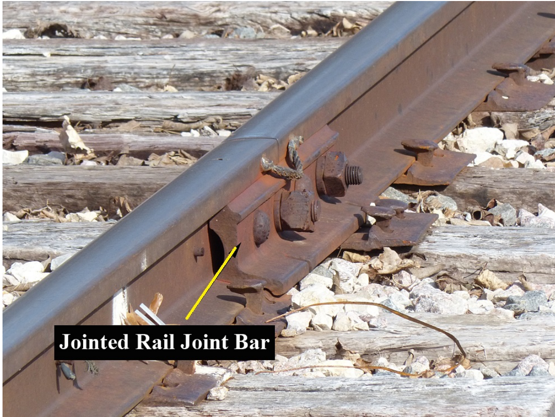
Figure 111: Jointed Rail Joint Bar 438
