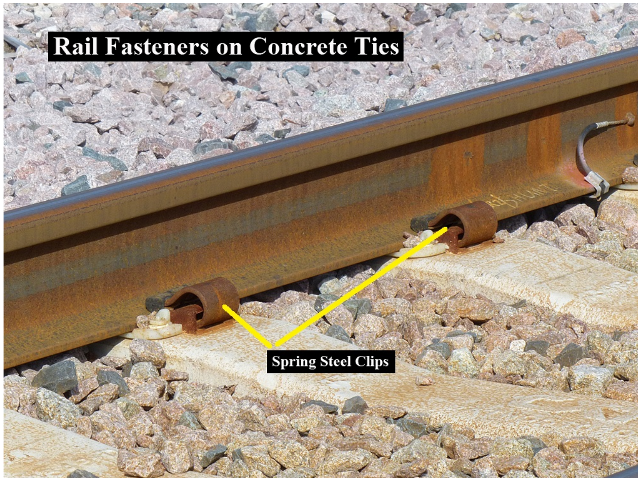
Figure 69: Rail Fasteners on Concrete Ties (Spring Steel Clips) 274
