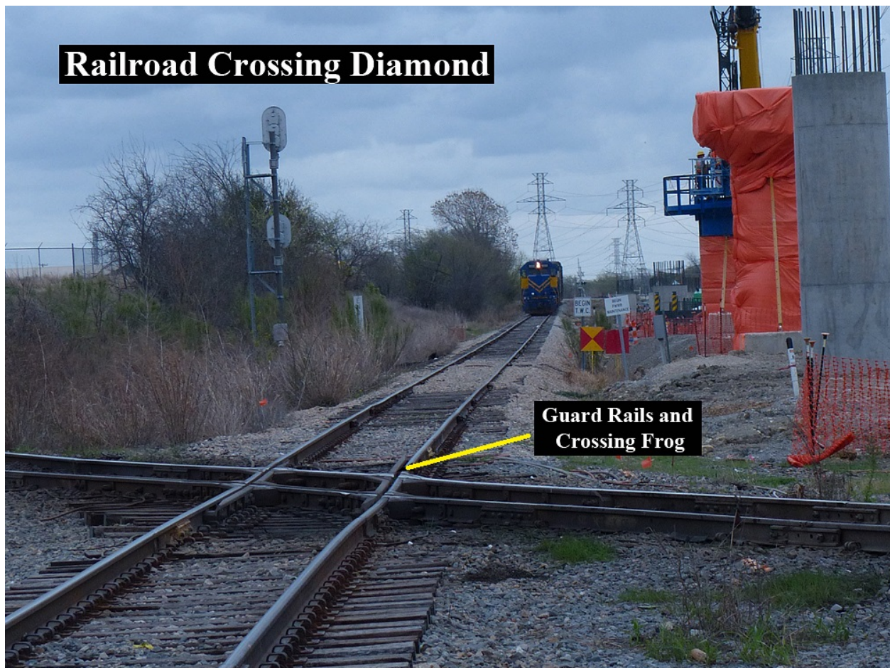
Figure 108: Railroad Crossing Diamond Showing Guard Rails and Crossing Frog 435
