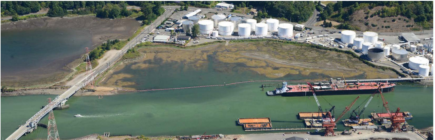
Regulated oil handling facility and vessel operating on the Hylebos Waterway, Tacoma, Washington.
