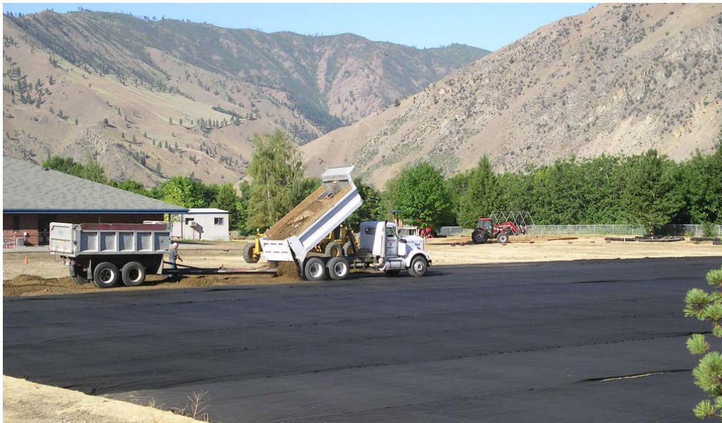
Contractors placing clean topsoil over geotextile fabric in redeveloped orchard lands. The topsoil and fabric act as a cap, keeping people safe from contacting lead- and arsenic-contaminated soil.
