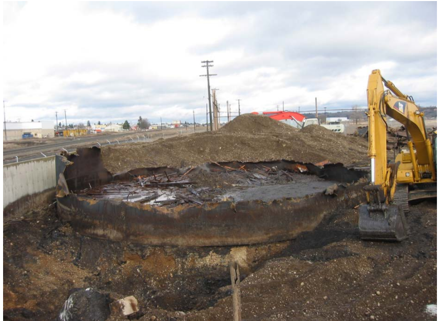
Black tank demolition, 2006.
