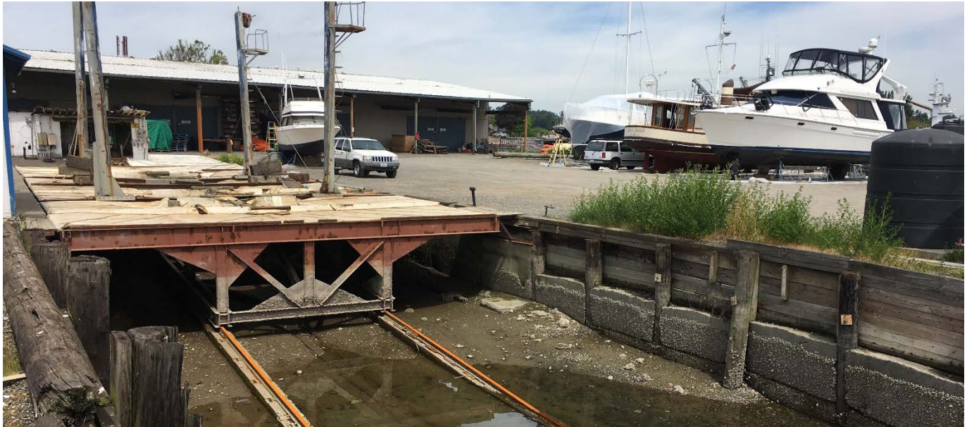
Westman Marine site marine railway and boat maintenance area
