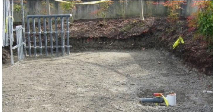
A soil vapor extraction system
