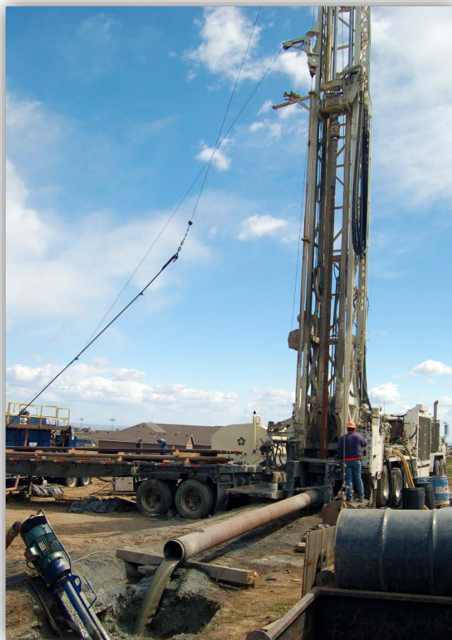
Test well drilling site, City of Kennewick
