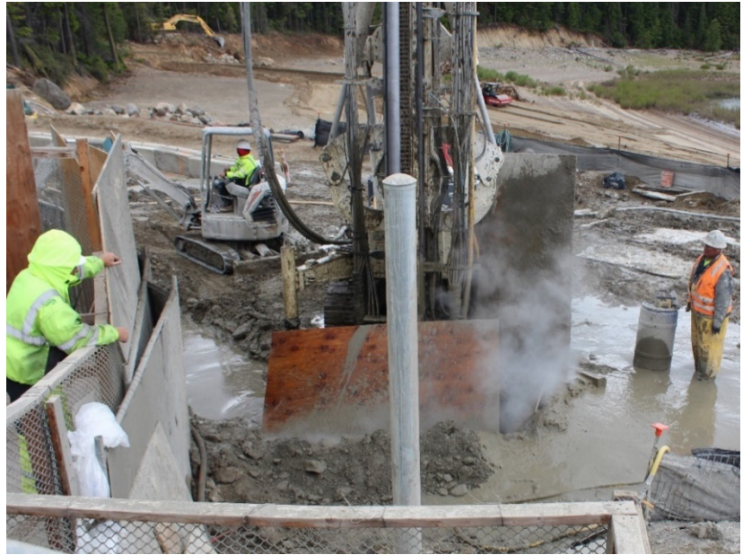
Cle Elum Fish Passage construction, June 2019
