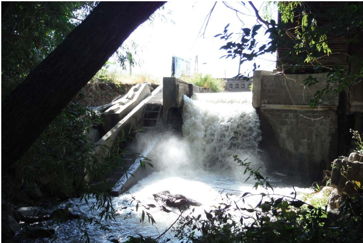
Figure 8. Wide Hollow Creek at the gravity drop located at the historical grist mill in Union Gap. The Alaska steep-pass fish ladder is to the left of the waterfall.
