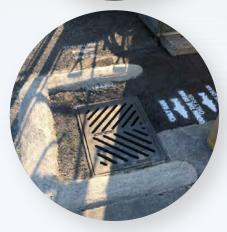
As a permanent solution, the facility installed a concrete berm around three sides of the storm drain. The facility also stenciled several storm drain labels next to the drain to educate people that only rain can go down the drain.
