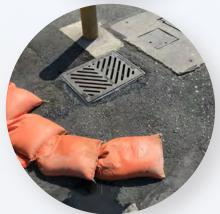
Specialists directed the marina to stop discharging wash water into the storm drain immediately and come up with a permanent solution. As a temporary solution, the facility added sand bags next to the storm drain to divert wash water away from the drain.
