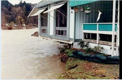
Cedar River flooding threatening mobile home park. The homes were purchased and removed, while the floodplain was reconnected.
