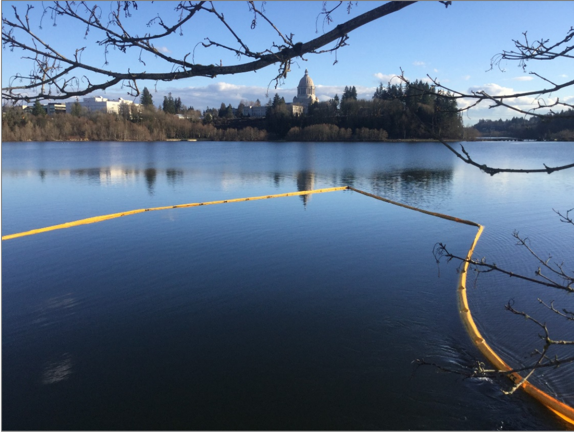
Figure 25: Deployed boom for the Olympia Brewery Transformer Spill
