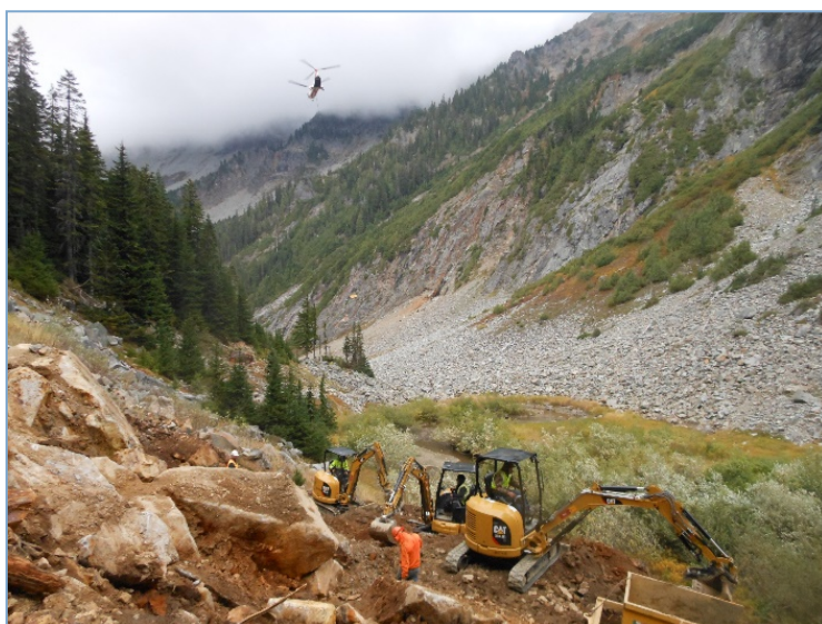
Figure 16: Excavation to divert mine water drainage from entering streams on the site.
