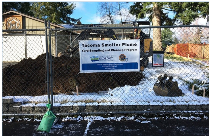
Figure 10: An Ecology contractor removes and replaces soil in a snowy yard in North Tacoma.
