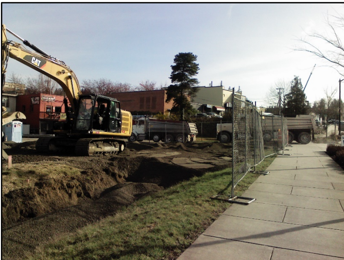
An interim cleanup action at the Bothell Riverside site.
