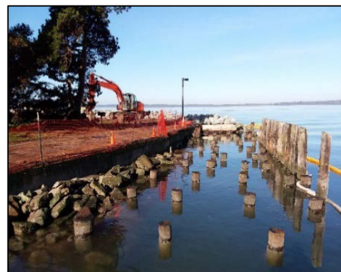
Public pier removal, October 2017
