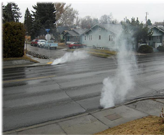
Figure 35: Illicit connection smoke testing.
