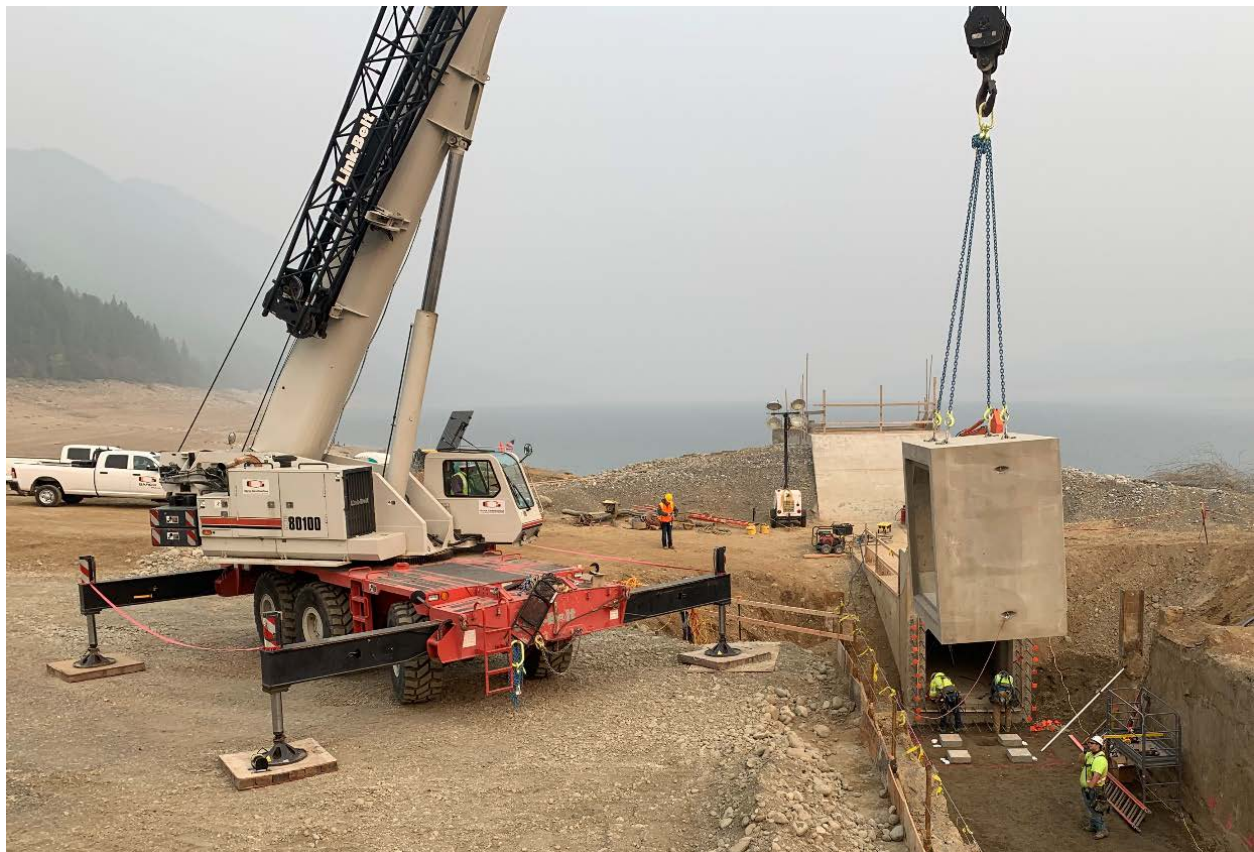
Installation of a juvenile fish intake ramp at Cle Elum Reservoir Fish Passage
