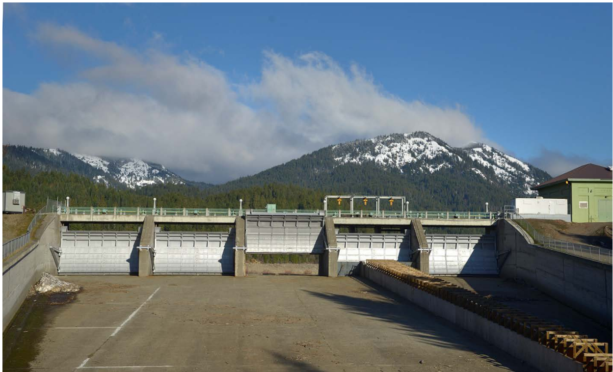
Cle Elum Dam Pool Raise Radial Gates
