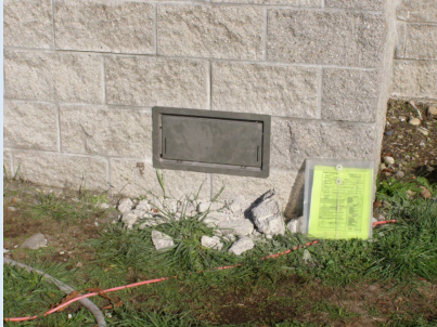
Engineered flood vent
