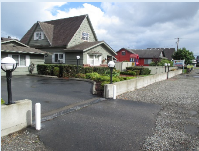
Local flood wall
