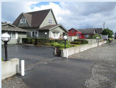
Local flood wall
