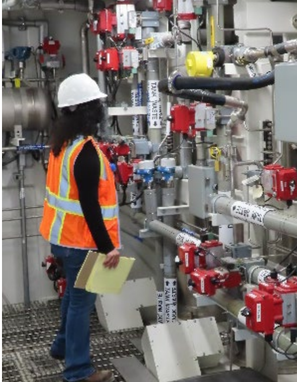
Nitya Chandran, a Waste Treatment Plant Facility Engineer for the Nuclear Waste Program, inspects part of the Tank-Side Cesium Removal System (TSCR) at Hanford. Ecology conducts frequent inspections at various Hanford facilities. TSCR is expected to begin treating tank waste in early 2022.
