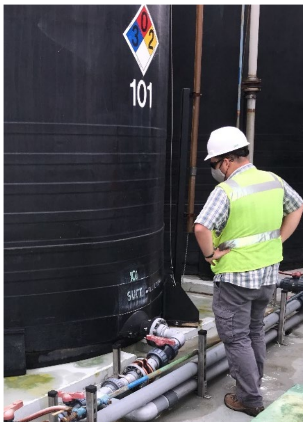
Engineer Jason Landskron inspects hazardous waste tanks at a business in Tacoma, WA.
