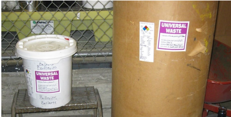
Figure 6: Properly labeled and closed containers of universal waste batteries and fluorescent tubes.
