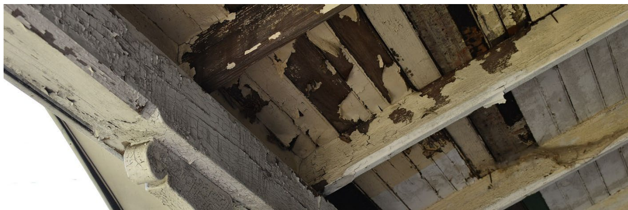
Figure 10: Lead-based paint can be a problem if it peels and cracks like this. Photo credit: Ich on Wikimedia Commons.
