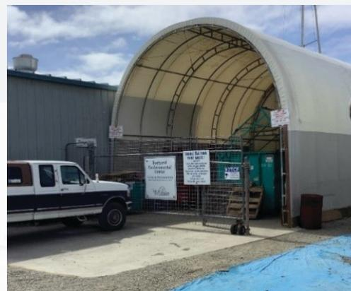
*Centralized oil collection location. Putting all the oil collection and management devices in one location lessens the impact from oil sitewide and means that there is only one place to worry about when it comes to oil management.*
