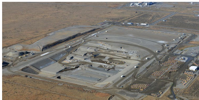
Figure 2 - Aerial View of ERDF - photo courtesy of DOE
