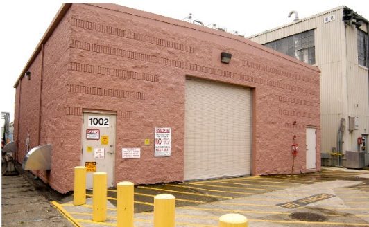
Figure 3 Exterior of MWSF
