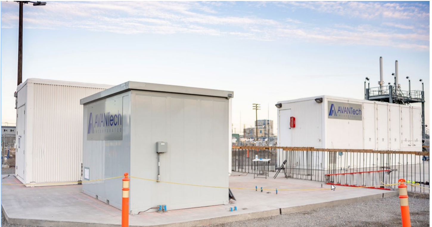
Figure 1 Process, Ancillary, and Control Enclosures on the Balance of Facilities pad- photo courtesy USDOE
