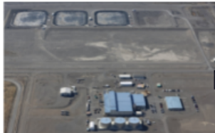
Hanford's Effluent Treatment Facility (ETF) is shown in the bottom part of this image, with the Liquid Effluent Retention Facility in the top portion. (Photo courtesy USDOD)
