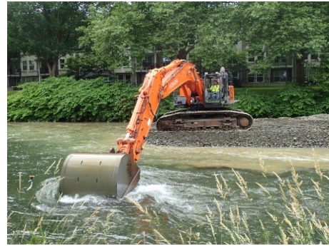
In 2016, the City of Renton dredged the lower 1.25 miles of the Cedar River to maintain adequate flood conveyance and protection. The permitting process, albeit rigorous, was aided by precedent as the work is a continuation of a Seattle District Corps Section 205 Flood Hazard Reduction Project initiated in 1997.
