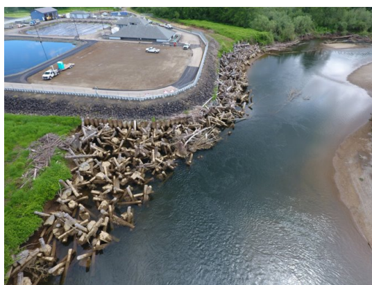
Engineered “log jacks” provide bank protection at the City of Montesano Wastewater Treatment Plant along the Wynoochee River in Grays Harbor County. Top photo is during construction, bottom photo is 1-year post construction. Note that the river angle of attack has shifted away from the facility.
