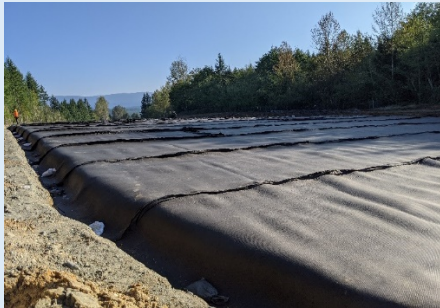
Partly completed trench cap, Landsburg Mine Site
