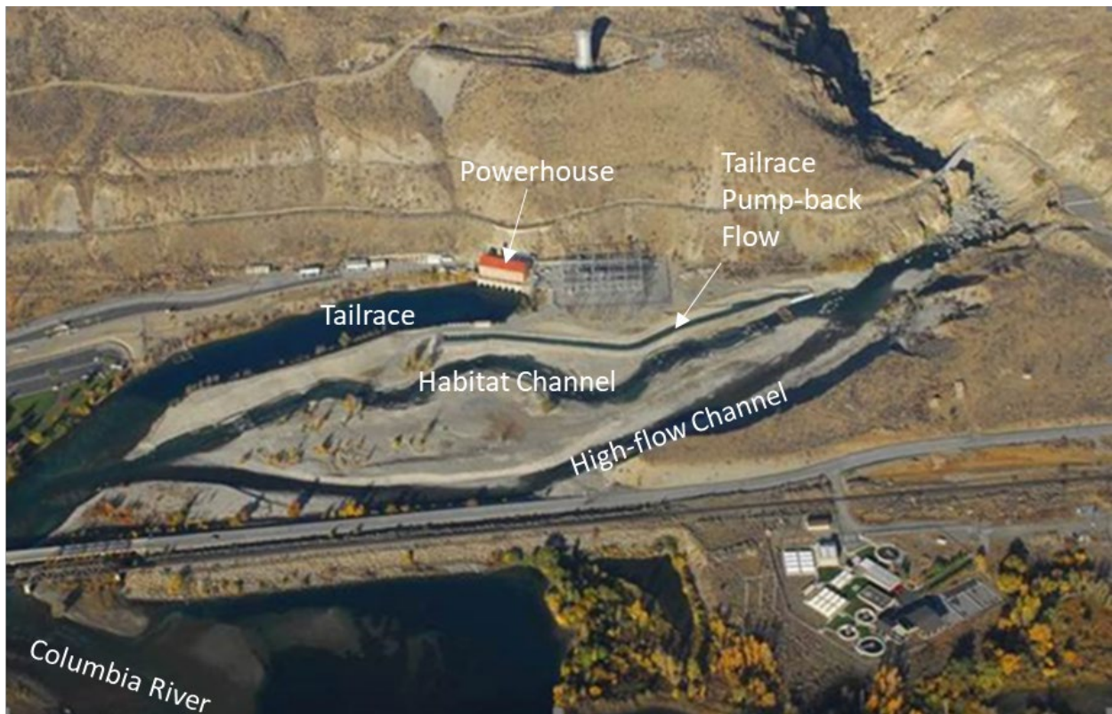
Figure 20 Reach 4 after restoration of instream minimum flows and the construction of the habitat channel in 2009 (adapted from Mugunthan et al. 2019).
