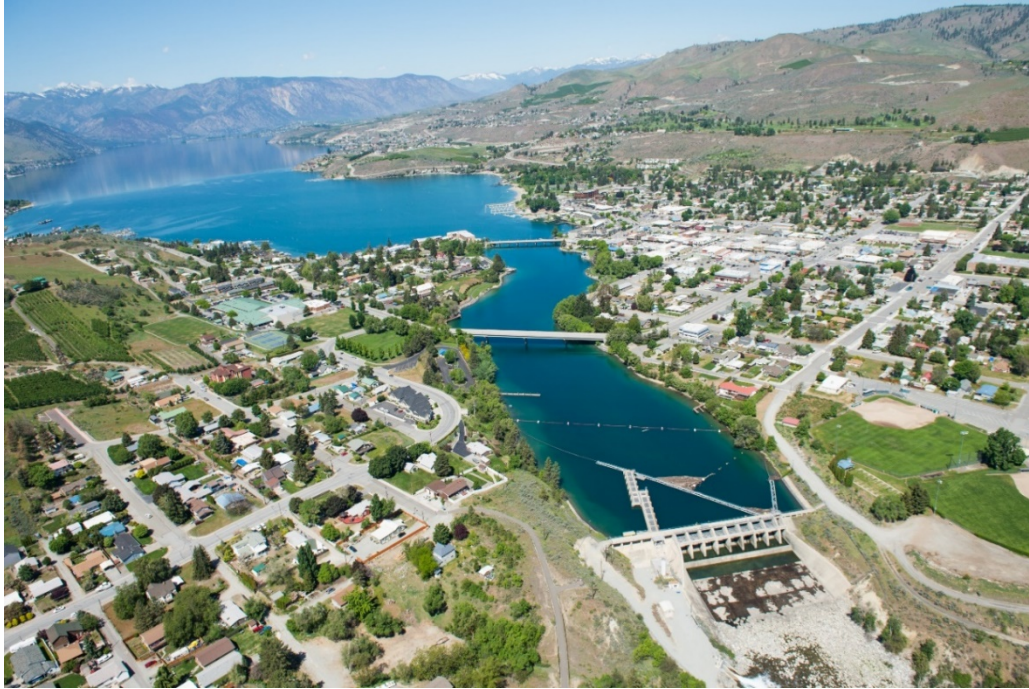
Figure 1 Lake Chelan and the Lake Chelan Hydropower Project at the headwaters of the Chelan River. Photo: Chelan PUD
