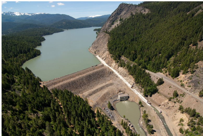
Aerial view of Tieton Dam
