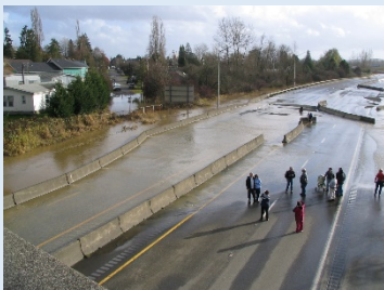
Catastrophic 2007 Basin flood closed I-5.
