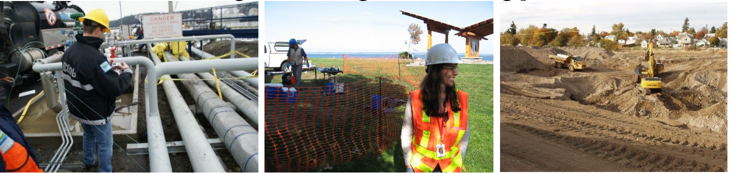
Figures 1 and 2: Ecology engineers surveying a job site.
