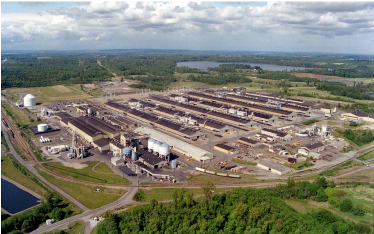
Figure 2. A bird's eye view of Intalco looking northeast across the facility toward Lake Terrell (source: https://nwcitizen.com/ )
