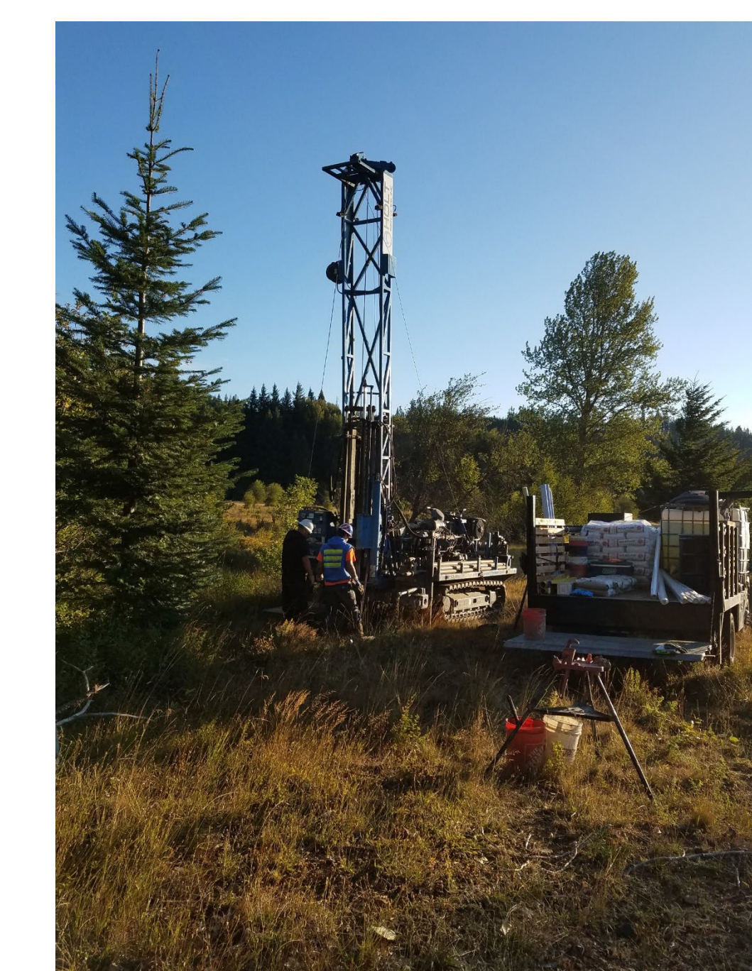
Drilling in Klickitat County
