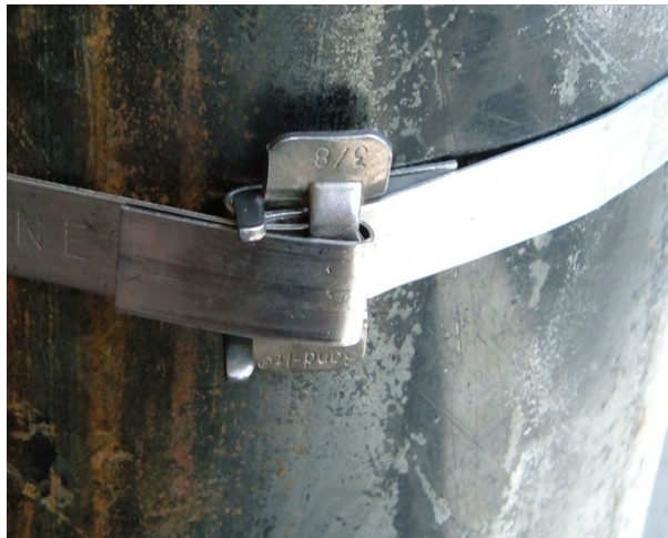
Figure 10. Locking the band.
