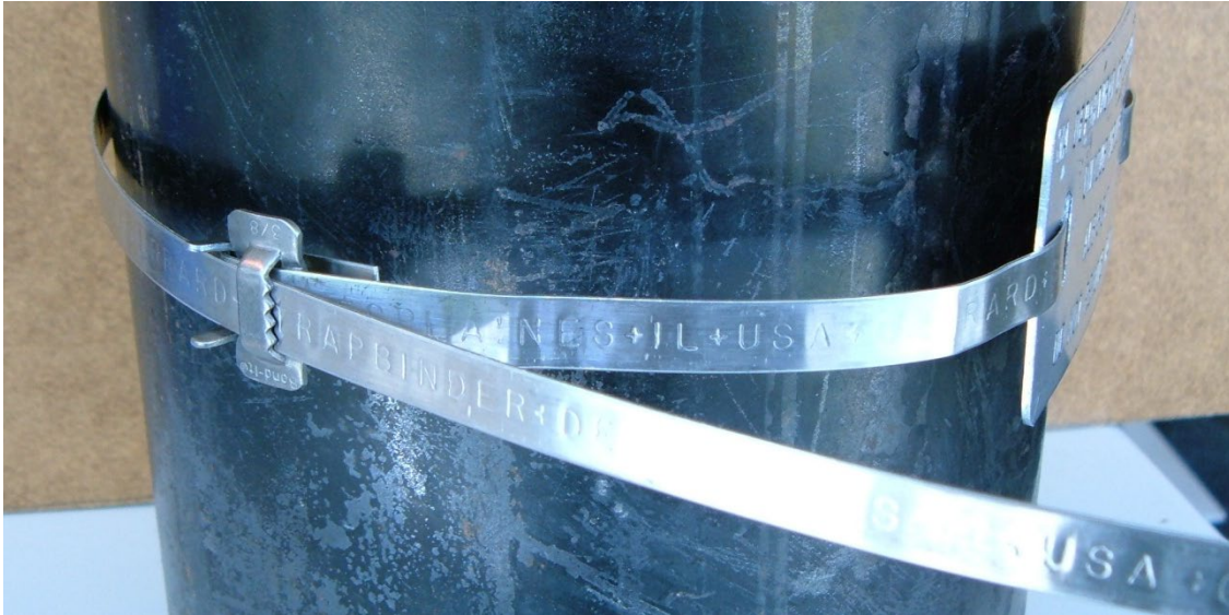
Figure 5. Wrapping the band around the well casing
