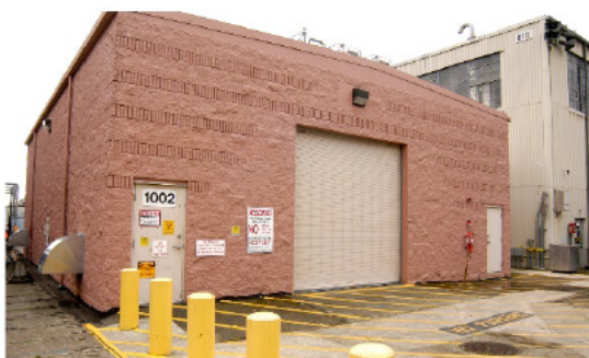
Figure 3 Exterior of MWSF
