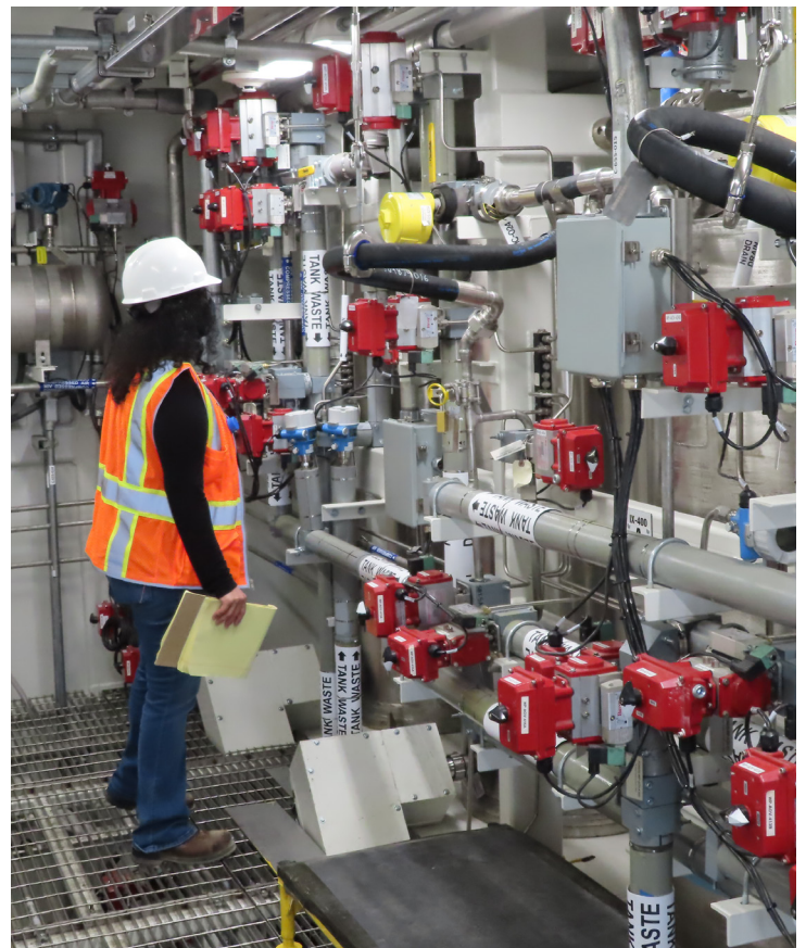
Ecology staff inspects the Tank-Side Cesium Removal system.
